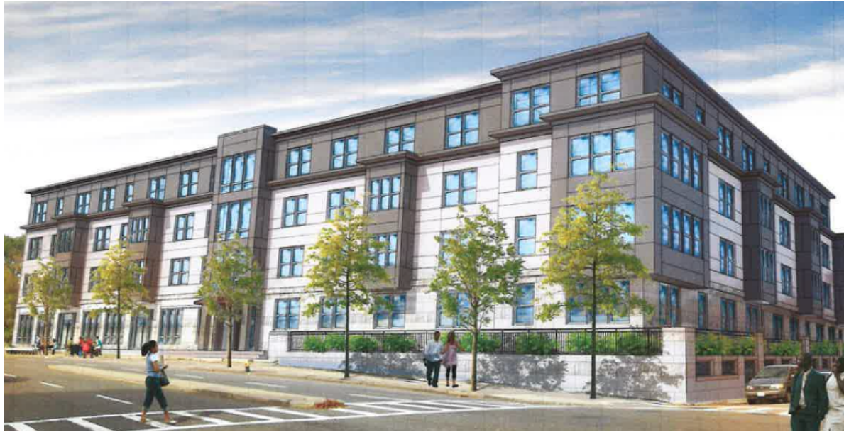
Cummins Highway Apartment Building
